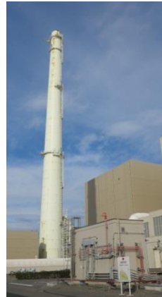
Vent stack common to Hamaoka Units 1 and 2
